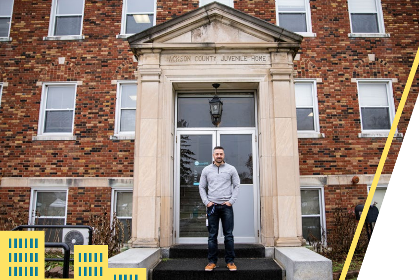
The old Jackson County Juvenile Home building now houses Rise Above.
